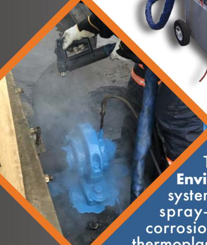
The **Enviropeel** system uses a spray-applied, corrosion-inhibiting thermoplastic coating to provide a tough, impermeable encapsulating barrier that prevents ingress and stops corrosion in its tracks.
